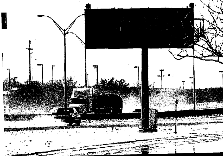
The new computer-based weather and road behavior system will suggest ways maintenance managers can address a specific problems, including determining appropriate chemical concentrations and application amounts, optimizing treatment times and strategies, and scheduling crews.
