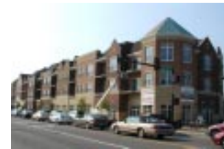
Varied roof forms and wall planes add interest to the building, and make them more comfortable to pedestrians walking along their facades
