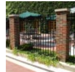
Urban gardens and garden-like edges to private spaces or parking lots offer spaces and objects of value to pedestrians
