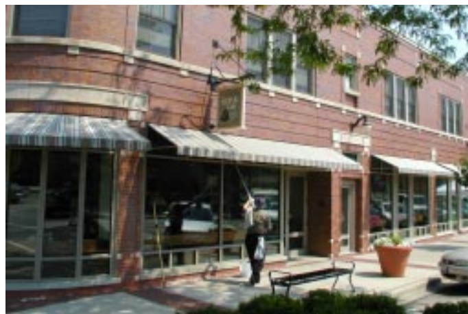
Awnings, traditionally used to block severe sunlight into storefronts, provide a certain level of protection from the elements for pedestrians, even if they are not continuous along a storefront
