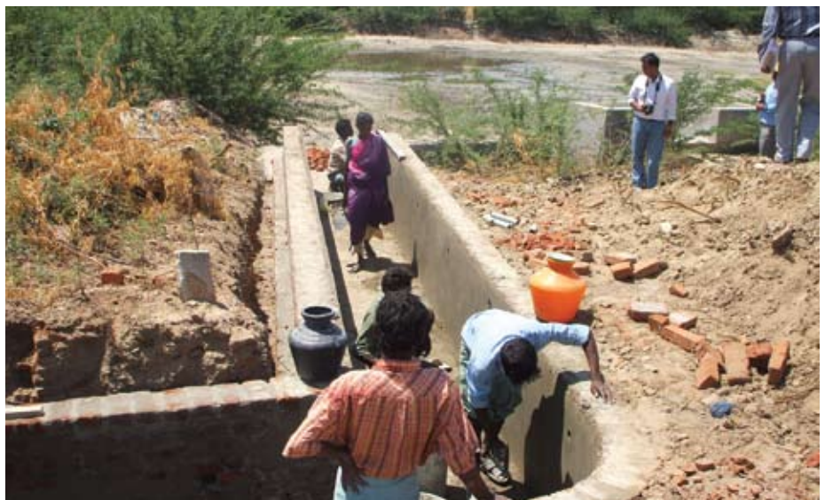
Ponds being interconnected in Nagapattinam to mitigate flooding.
