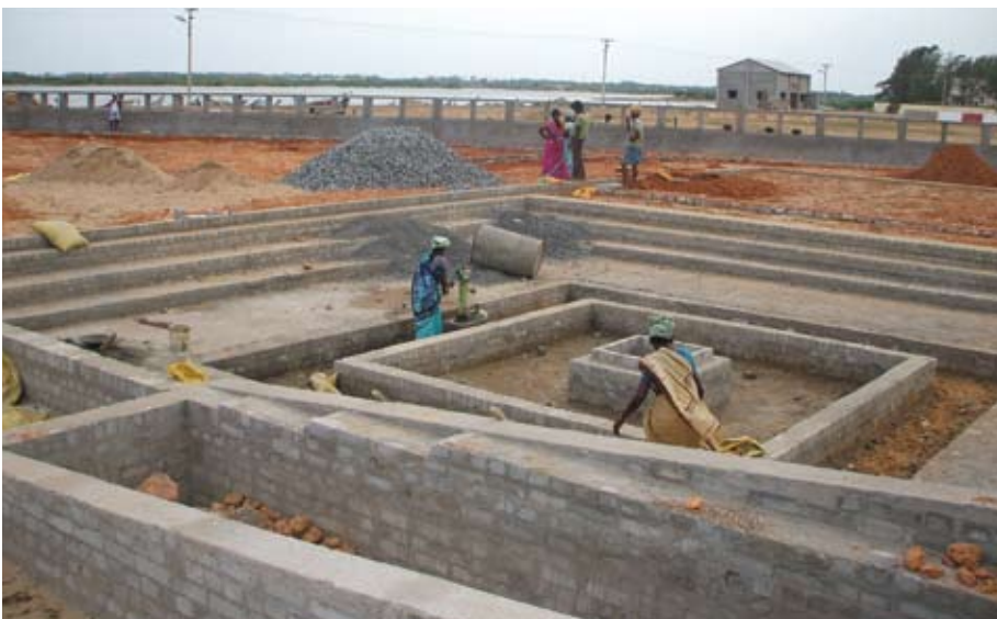
Park construction on Silver Beach in Cuddalore.
