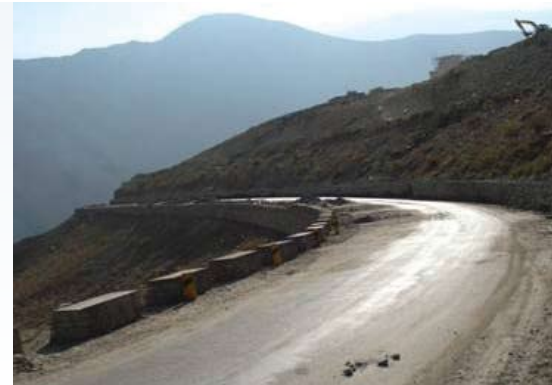
Near Bazarak, the capital of Panjshir province, the CityLinks team eliminated a significant roadway hazard by building this safety wall at a dangerous curve along an important transportation route.
