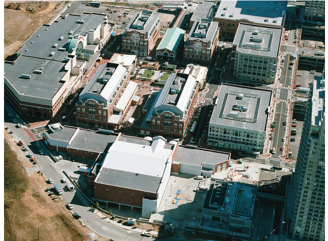
Atlanta's Atlantic Station is a successful example of infill development. Residents of Atlantic Station drive less than half as much as residents in other parts of the Atlanta Metropolitan Area.
