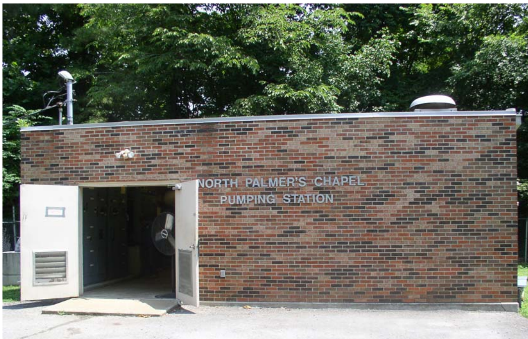
Figure 4.3 – North Palmer's Chapel Vacuum Pumping Station
