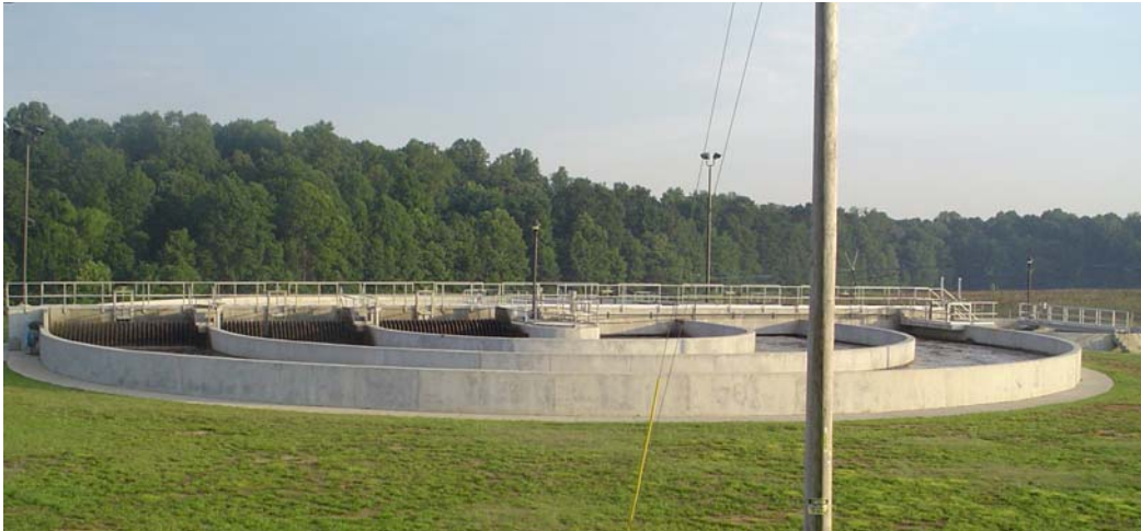
Figure 4.24 – WWTP – Oxidation Ditches
