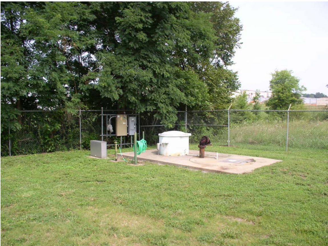
Figure 4.21 – Springfield Lift Station
