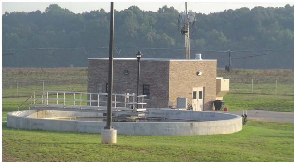
Figure 4.25 – WWTP – Secondary Clarifier and RAS/WAS Pumping Station
