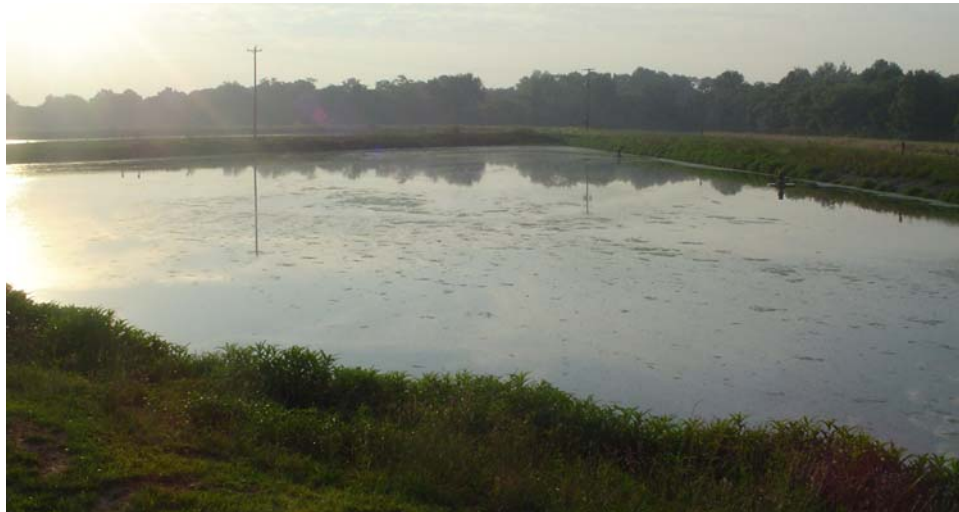
Figure 4.26 – WWTP – Aerated Lagoons
