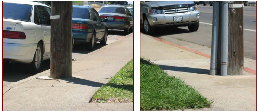
Figure 3: Utility Pole Obstruction Examples - Mather Field Road at the Mather Sports Complex and Senior Center
