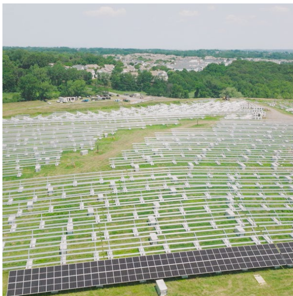
Aerial shot of the Old Bridge at the AC Power site.
