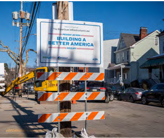
Lead pipe replacement, Pittsburgh, Pennsylvania
