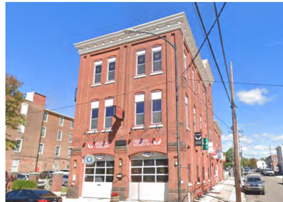
Five Saints Distilling redevelopment, Norristown, Pennsylvania
