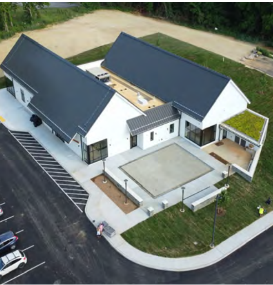
Shepherdstown Library redevelopment on former landfill, Shepherdstown, West Virginia
