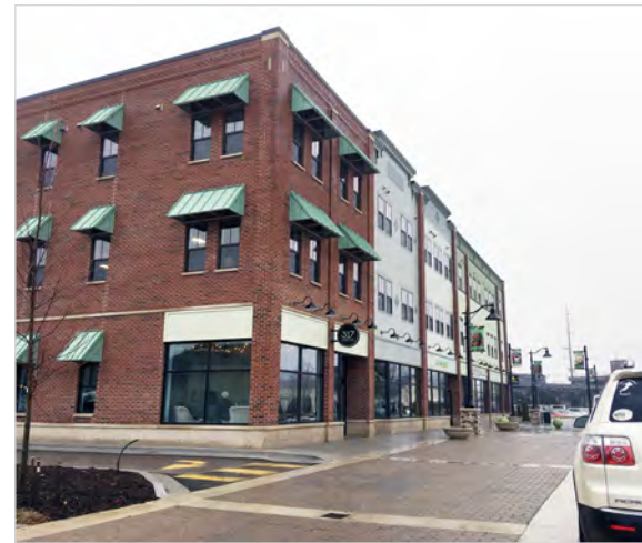
Completed Hudson Center redevelopment, Hudsonville, Michigan
