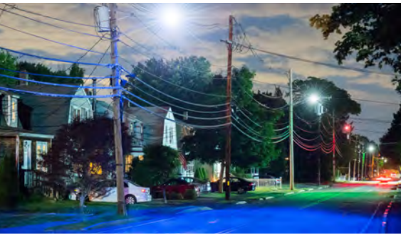
Colored streetlights installation, Ashland, Massachusetts
