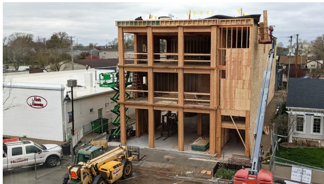
West Valley Junction New Construction
