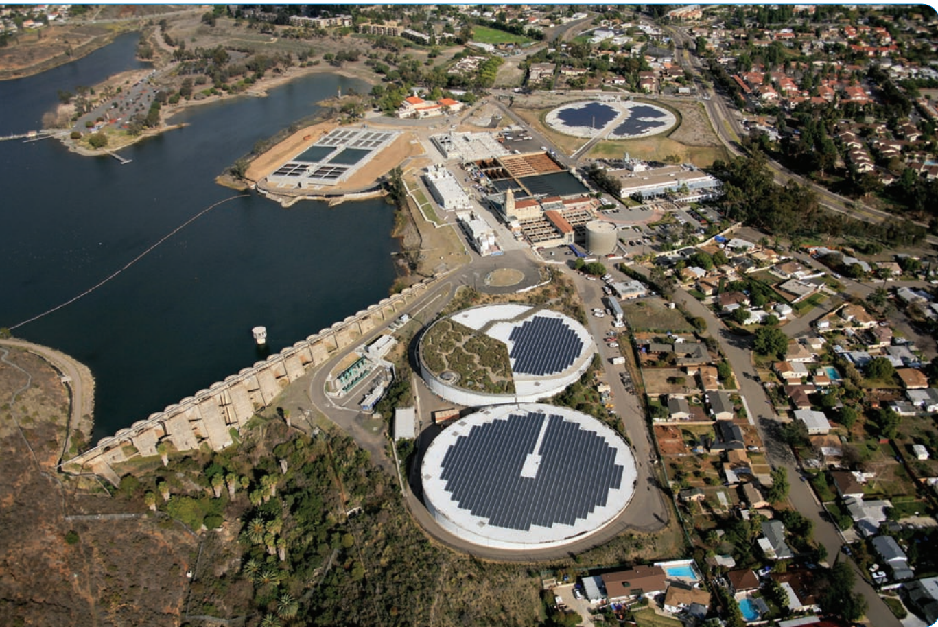
San Diego Alvarado Water Treatment Plant (Photo credit: SunEdison)
