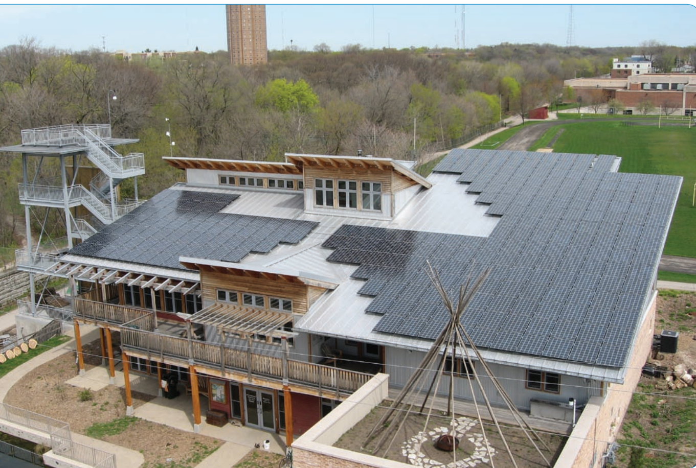
PV panels on Milwaukee, Wisconsin's Urban Ecology Center. (Photo credit: Urban Ecology Center)
