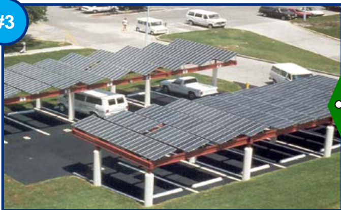
Parking Structure Solar PV
