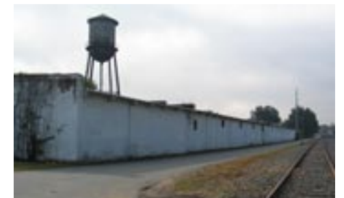
Anchor Mill property
