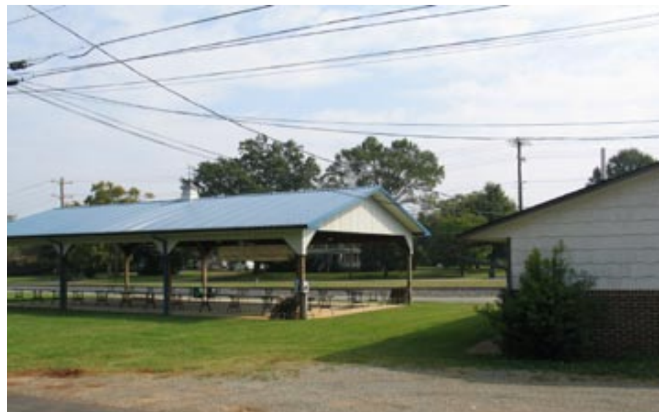
Current view of Farmer's Market shelter
