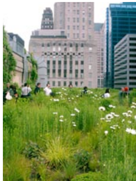
Planted roofs minimize stormwater runoff and reduce heat gain like this one on the Chicago City Hall
