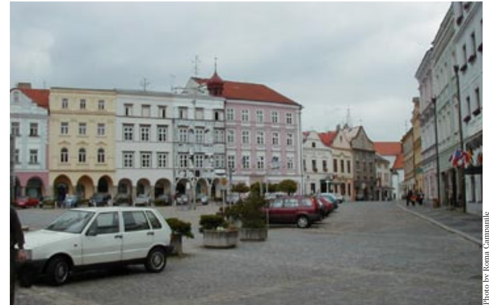
European plaza where pedestrians have an equal footing with the car
