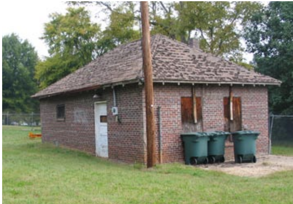
Existing condition of the "Old Jail"
