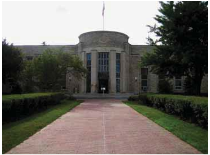
Saginaw City Hall. As a result of its strategic operation review, the city realized $3 million in annual recurring cost savings the first year. Photo by Junko Kimura.
