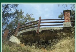
This project repaired the slopes along San Ramon Creek that were severely eroded by the winter storms of 2002, threatening to undermine the roadway approaches to the bridge. The project also beautified West El Pintado, incorporating a park-like setting at this gateway to the neighborhood. CIP #C-457.
