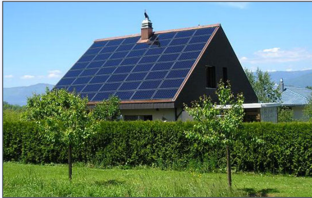
Solar Photovoltaic (PV)
