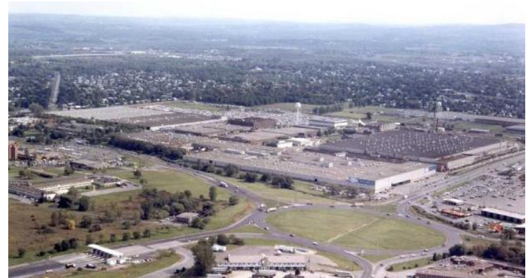
EXISTING SITE CONDITIONS
