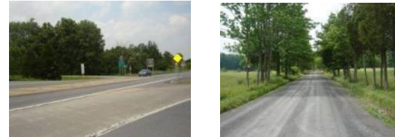
EXISTING SITE ENTRANCE
