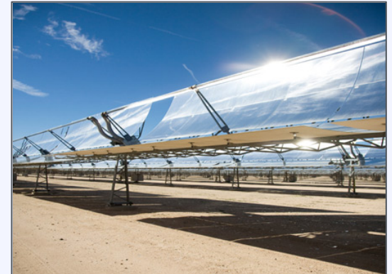
Concentrated Solar Power
