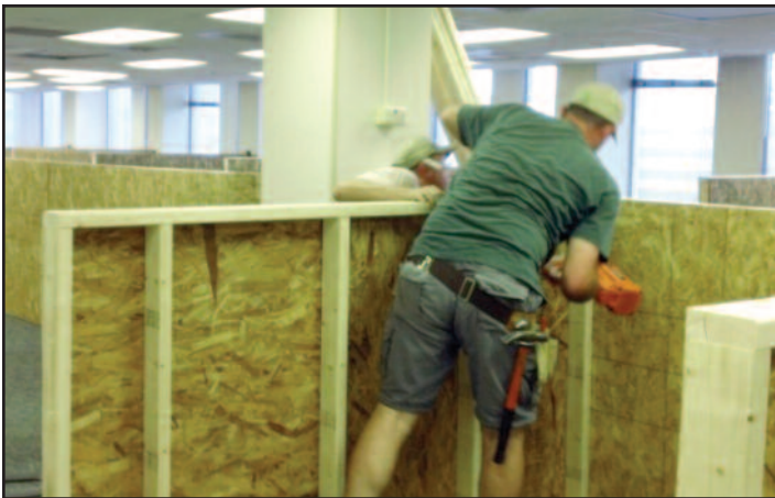
Figure 2: Office cubicle props on fire floor (10th)
