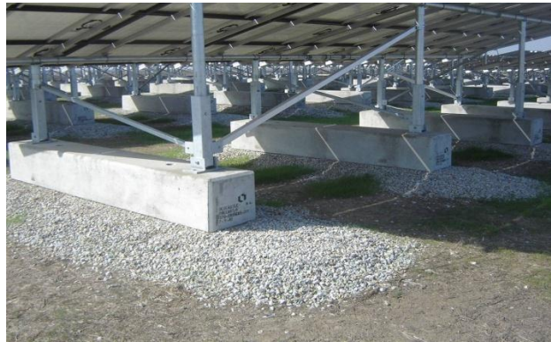
Figure 5-1: Precast ballast foundation for fixed tilt PV on a landfill
