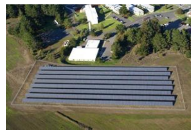
Source: NREL PIX 17395
