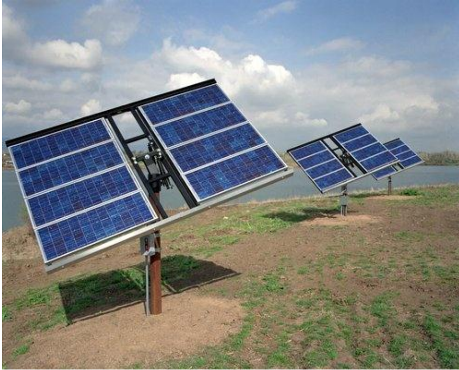
Figure 3-8: PV system with dual-axis trackers
