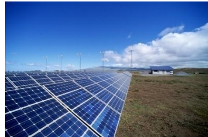
Source: NREL PIX 13823
