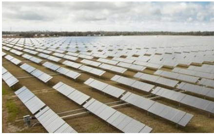
Source: SunPower Corporation
