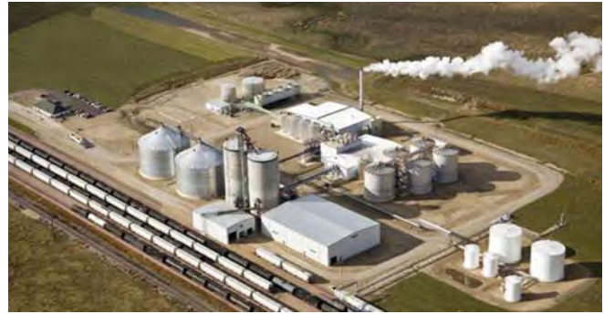
Bushmills Ethanol Plant located in the City of Atwater in Kandiyohi County, Minnesota. Photo courtesy of the Kandiyohi County EDC.
