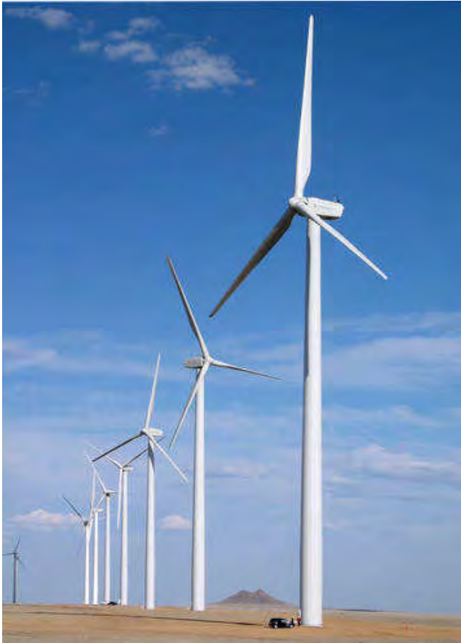
At the time of its construction in Prowers County, the Colorado Green Wind Energy Project, which has 108 1.5 MW wind turbines was the largest wind farm in Colorado and one of the largest in the country. Photo courtesy of Prowers County Economic Development, Inc.
