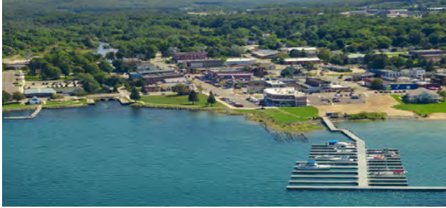
The expansion of the marina, resulting from the partnership between the developer and the city, has made it possible for more and larger boats (up to 147 feet) to dock in Boyne City. From the marina, nearby restaurants, shops, and a farmer's market are all accessible on foot, attracting activity to the area by both land and water. Photo courtesy of Boyne City.
