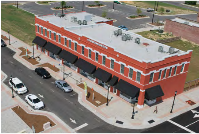
The Douglas Block after construction. Photo courtesy of the City of Rocky Mount.
