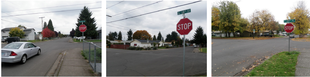
Figure 27: Turning the stop signs facilitates the flow of bicycles through the boulevard, and redirects vehicle traffic from entering the street.
