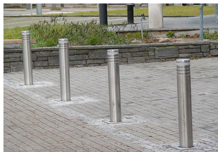
Figure 18: Remotely Retractable Bollards.
