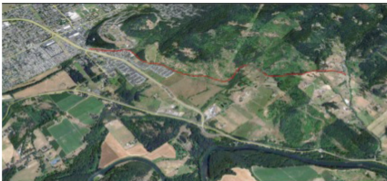
Figure 17: Aerial view of site area.
