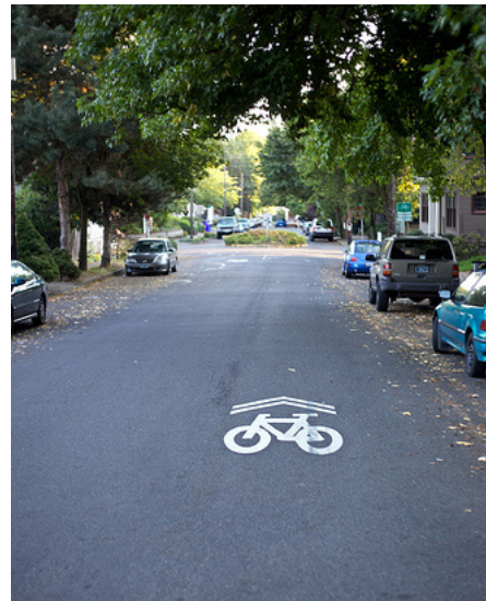
Figure 28: An example of what a sharrow might look like on Daisy Bicycle Boulevard.
