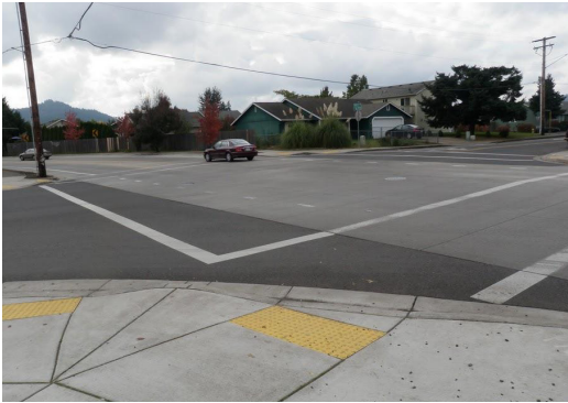
Figure 30: Current conditions at 42nd Street and Daisy Street.
