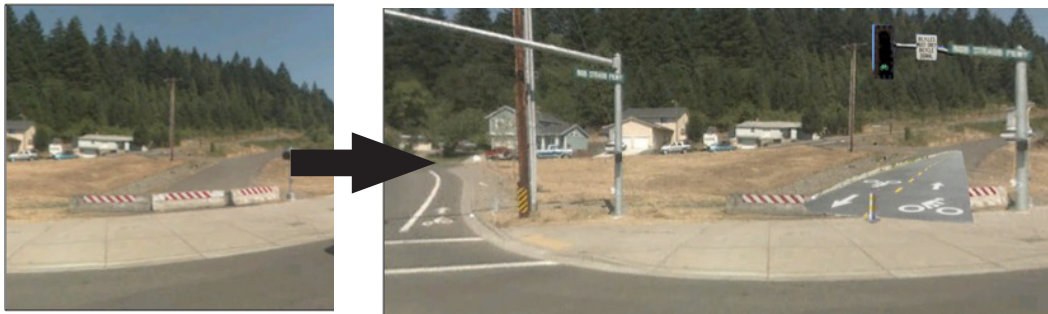
Figure 24: What the intersection would look like before and after the installation of a bicycle-crossing light.
