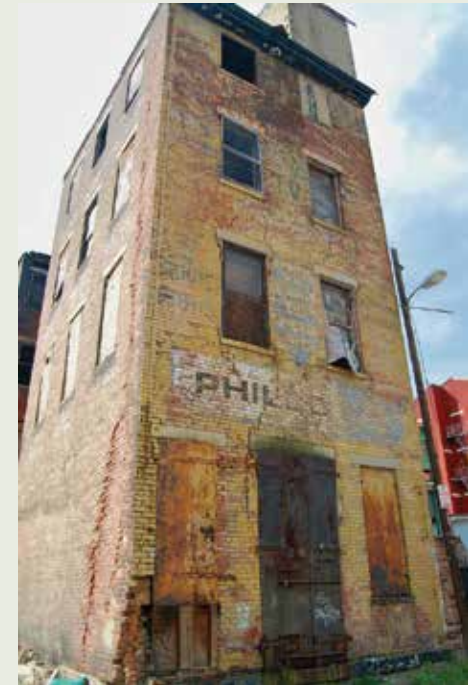
An abandoned commercial property in Cincinnati, Ohio.
