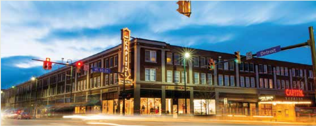
The restoration of the 1920s-era Capitol Theatre is a cornerstone of the revitalized Gordon Square Arts District in Cleveland's Detroit Shoreway neighborhood.
