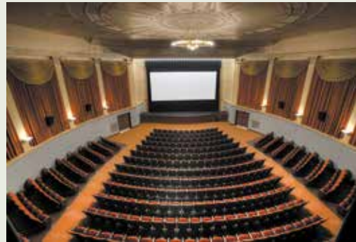
The auditorium of the Capitol Theatre after renovation by Marous Brothers Construction. Multiple funding sources were used to fund the redevelopment of the Capitol into an independent movie theater, including state capital funds.
