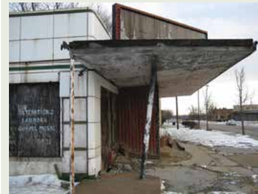
A vacant commercial building in Youngstown.
