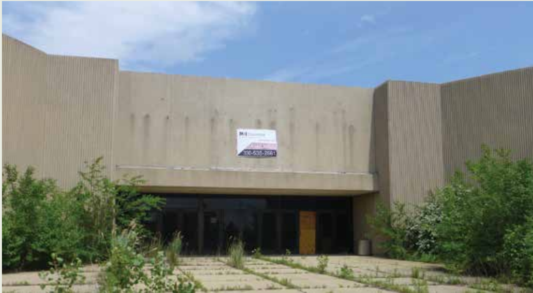
The May Company, a long-vacant department store in North Randall, Ohio.
