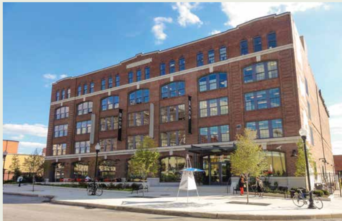
The redeveloped Maryland Institute College of Art (MICA) building in the Station North Arts and Entertainment District of Baltimore.
