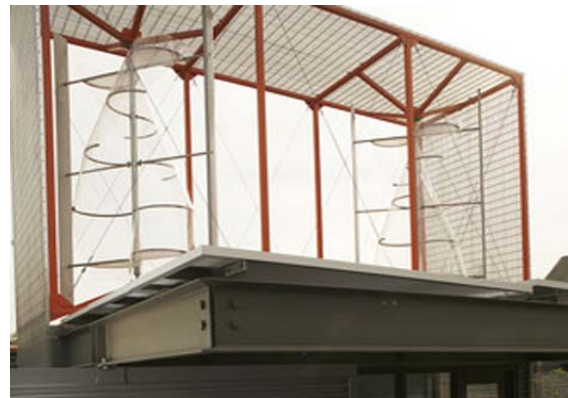
WIND TURBINE GENERATORS; MAUCERI RESIDENCE, CHICAGO
