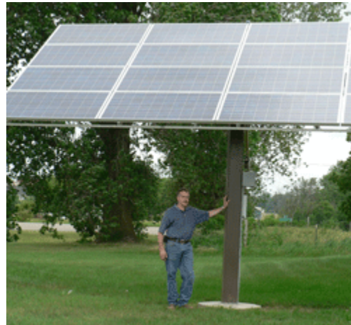
Figure 1: A 2.6 kW array installed at a local plumbing and electric shop. The system provides 25% of the shop's electricity (photo courtesy of RFMU).
