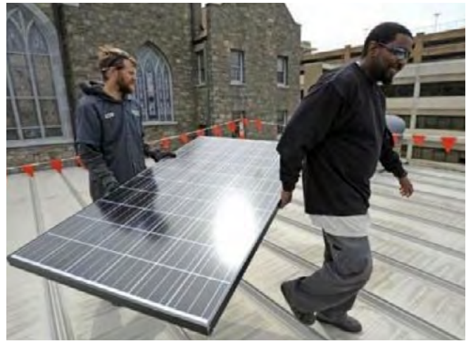
Solar panels are installed on First Congregational United Church of Christ
