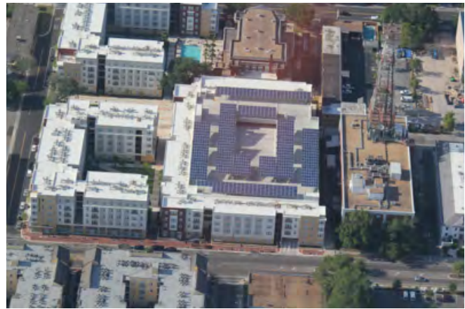
A 250-kilowatt solar installation undertaken through a third-party lease on the roof of an apartment complex for graduate students. The photovoltaic panels also provide covered parking on the top floor of the parking garage. Photo courtesy of Power Production Management.
