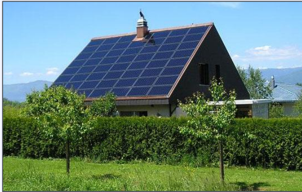
Solar Photovoltaic (PV)
