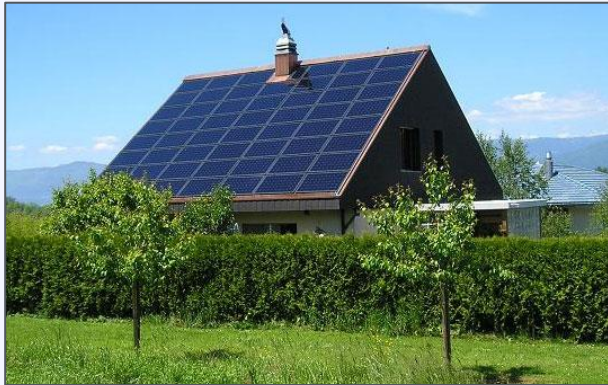
Solar Photovoltaic (PV)
