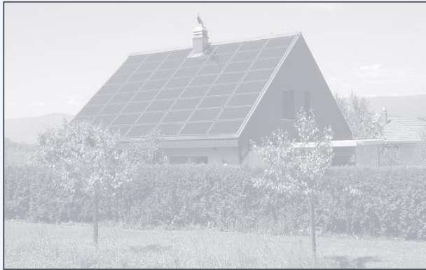
Solar Photovoltaic (PV)
