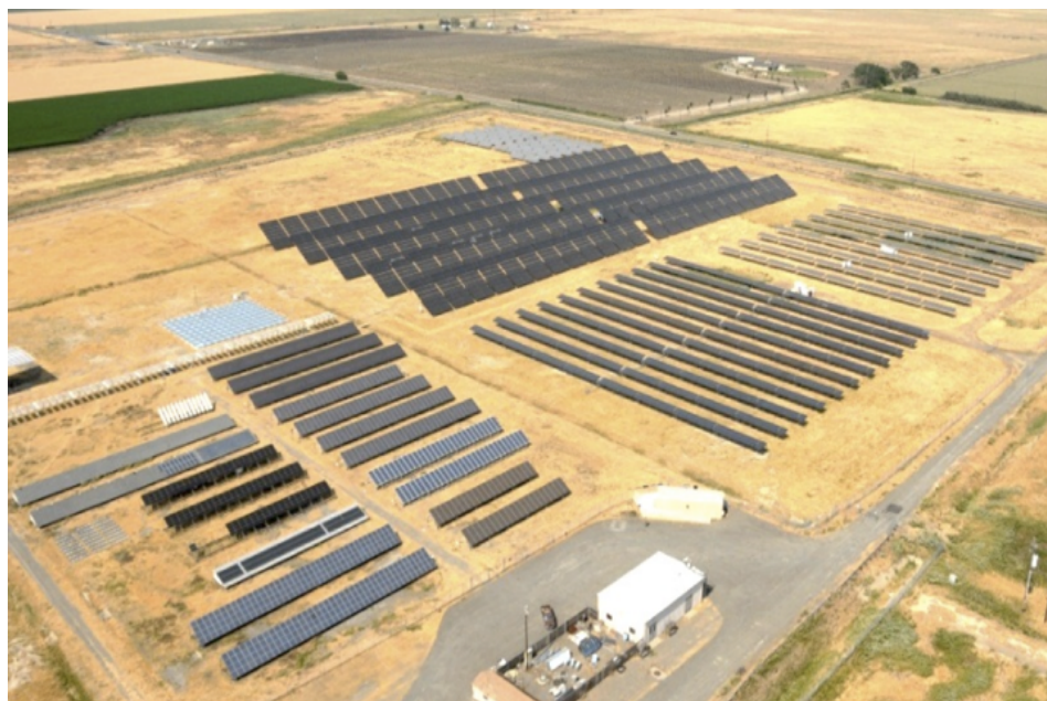
PV USA, a 1MW community solar project in Davis, CA
