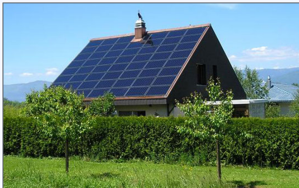
Solar Photovoltaic (PV)
