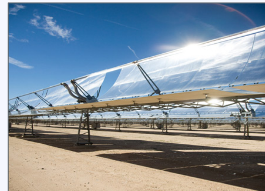
Concentrated Solar Power
