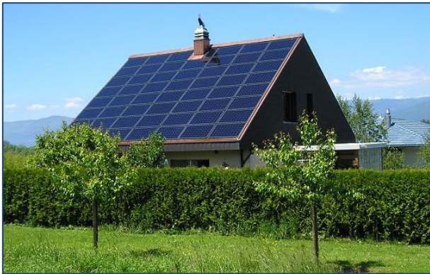
Solar Photovoltaic (PV)
