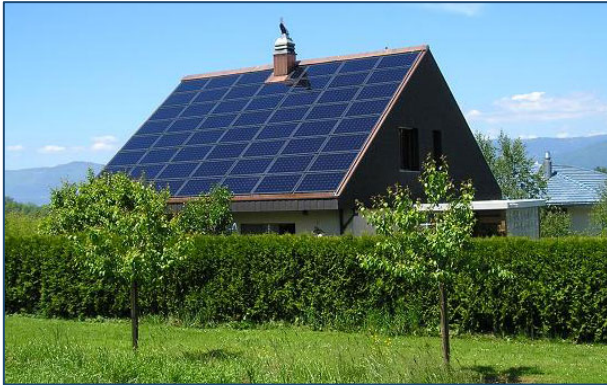
Solar Photovoltaic (PV)
