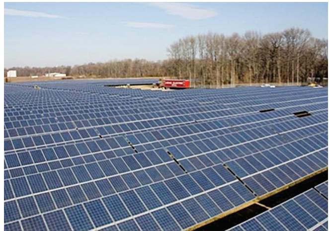
819 KW solar array at Water Pollution Control Facility.
