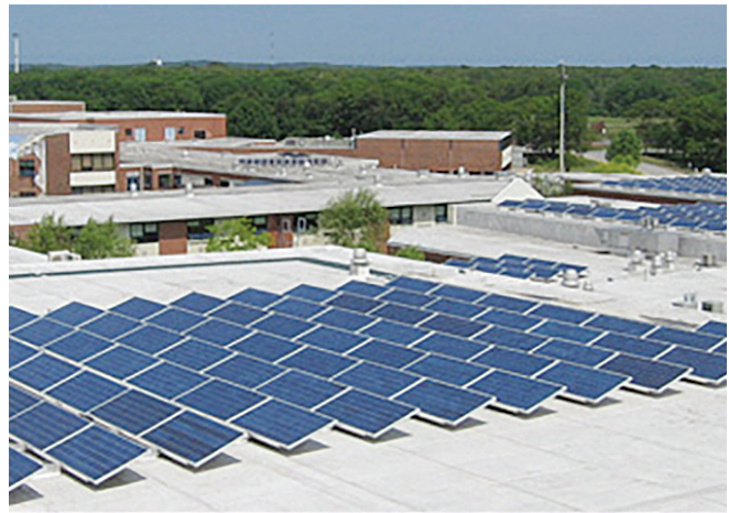
133 kW solar array at Barnstable High School.
