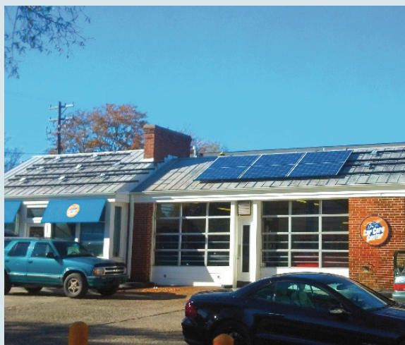
Chapel Hill Tire Care Company’s rooftop solar PV system.
