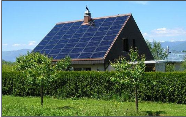
Solar Photovoltaic (PV)
