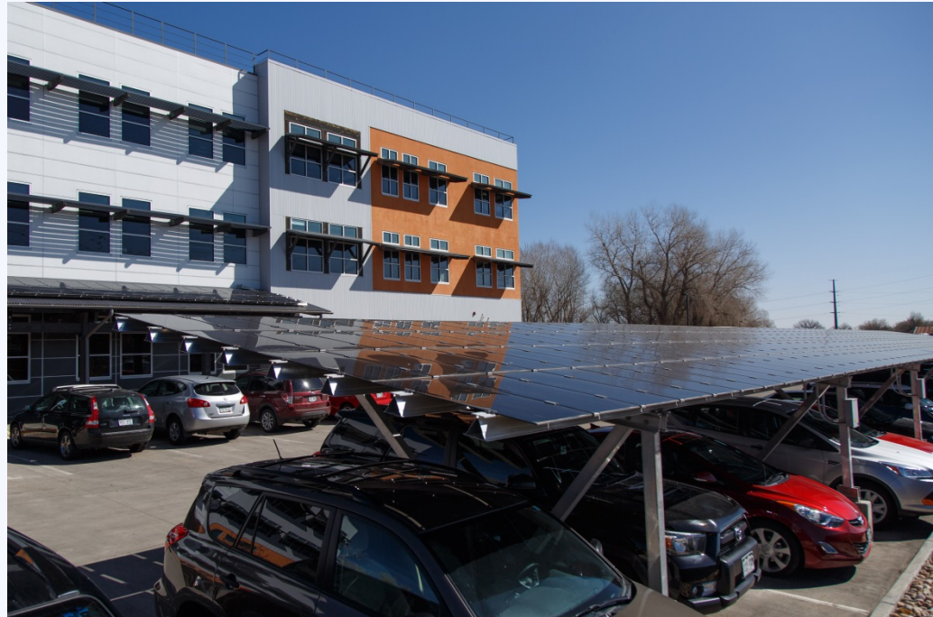
Solar carport structure and colors match building architecture
