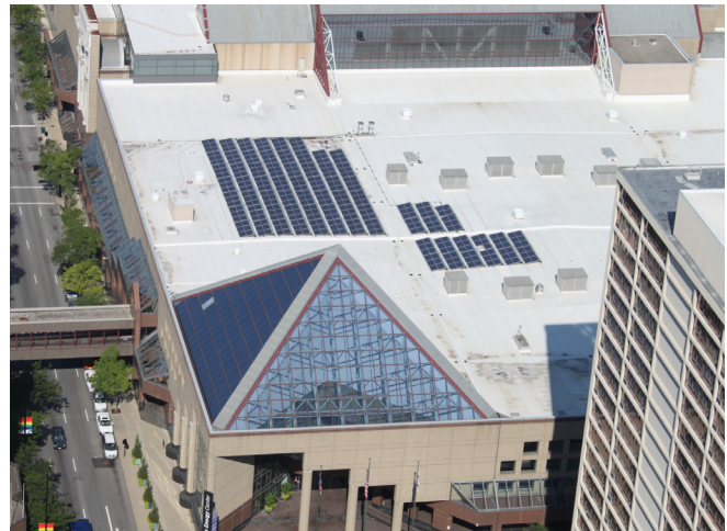
Aerial of the Solar Array on the Duke Energy Convention Center
