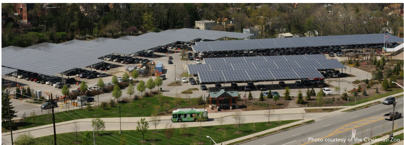
Aerial of the 1.6 MW Solar Parking Canopy at the Cincinnati Zoo
