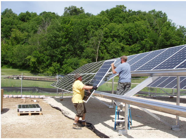
PV panel installation at WWTP
