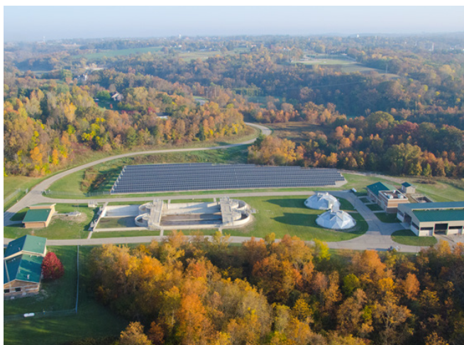
Aerial image of solar installation at WWTP
