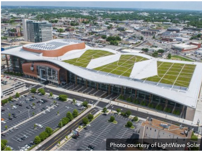
The green and solar roof of the Music City Center
