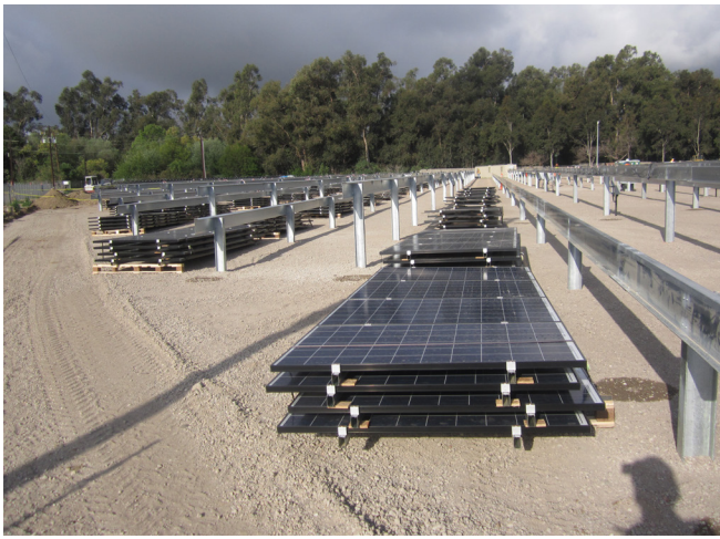
Solar panels ready for installation.
