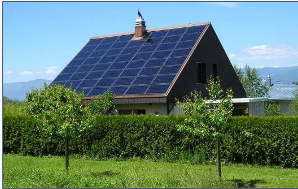
Solar Photovoltaic (PV)
