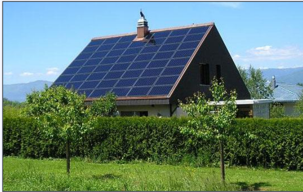
Solar Photovoltaic (PV)
