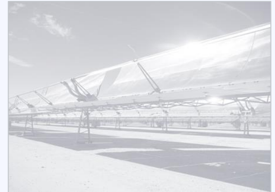
Concentrated Solar Power
