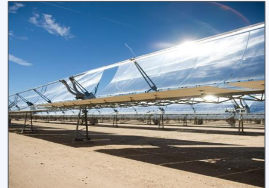
Concentrated Solar Power
