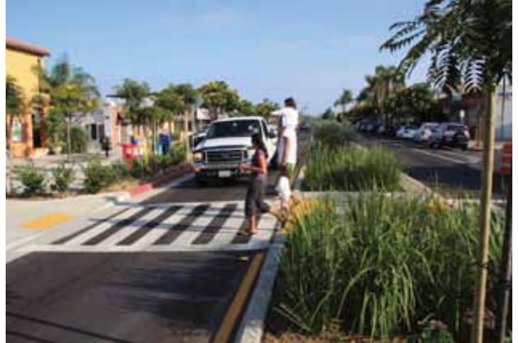
This roadway approaching a roundabout in San Diego, Calif., reduces the distance people must cross.
