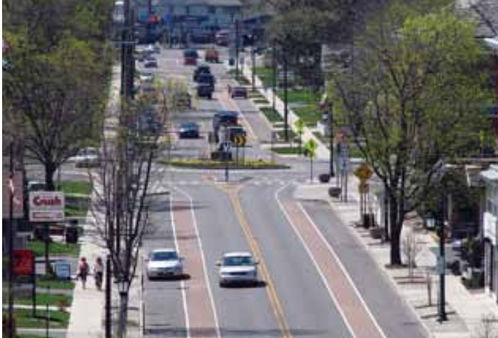
In Hamburg, N.Y., a series of roundabouts on Route 62 helps calm traffic and create a sense of place.
