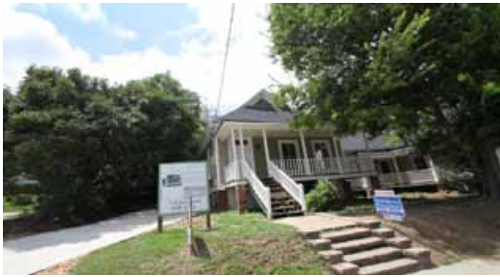
Preserved housing in Tattall Place, Macon, Ga., is part of a mixed-income redevelopment project.
