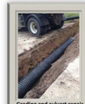
Grading and culvert repair
