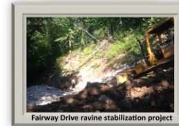
Fairway Drive ravine stabilization project
