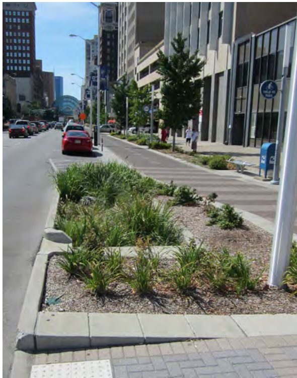
STORMWATER PLANTER INSTALLATION 5
