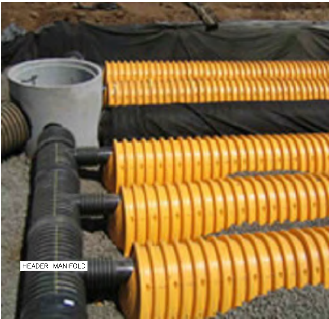
STORMTECH SUBSURFACE CHAMBERS ARE AN EXAMPLE OF UNDERGROUND STORAGE 3
