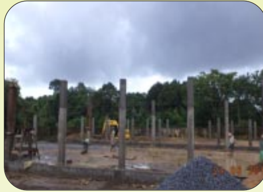
Vermi Compost Yard
