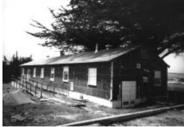
Demonstration for asbestos removal
