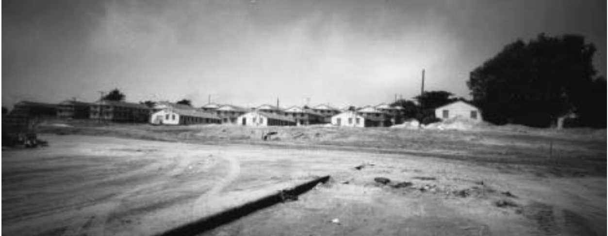
Building deconstruction and relocation cleared the way for the 12th Street Realignment
