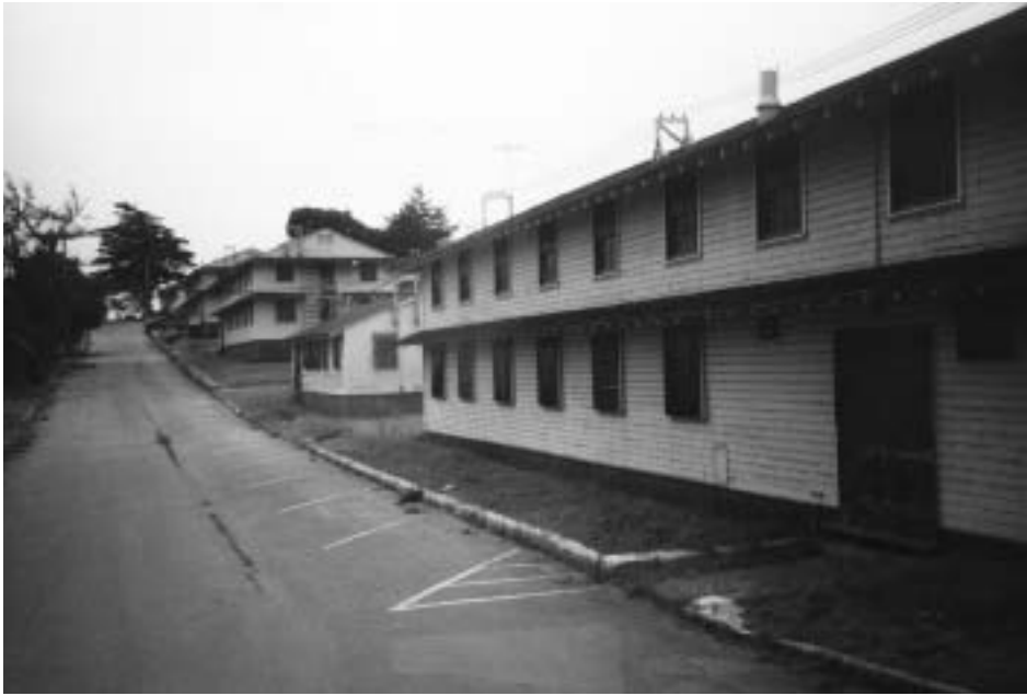
Rows of Army barracks contaminated with LBP and ACM
