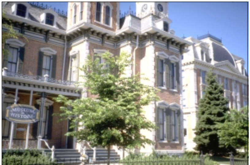
An accessible side entrance was added to this historic facility.
